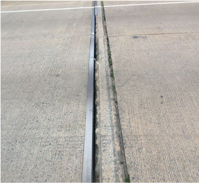
PHOTO 1 Description Joint armor missing at bent 5
