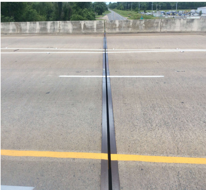
PHOTO 1 Description Bent 2 joint seal has fallen out.
